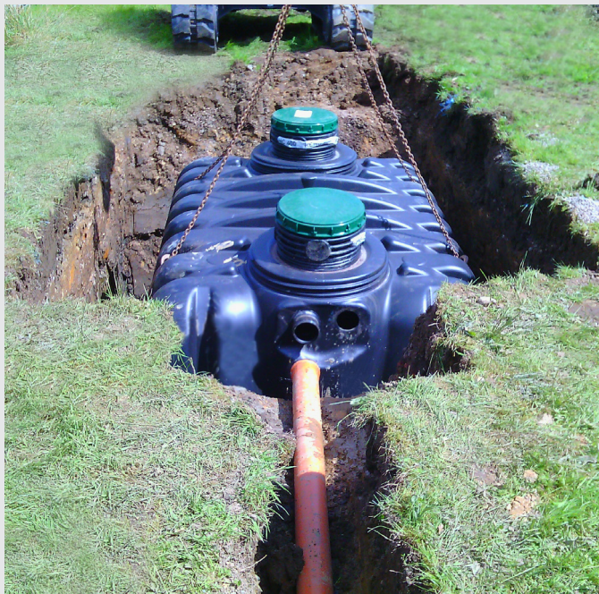
Tricel Vento installed.
