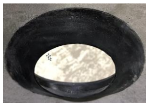
Inside of grommet fitted.
